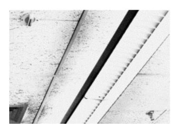
Typical <u>ceiling installation</u> of a horizontal DETECT-A-FIRE model. Here it is used in combination with a sprinkler system to detect overheat and actuate an alarm.
